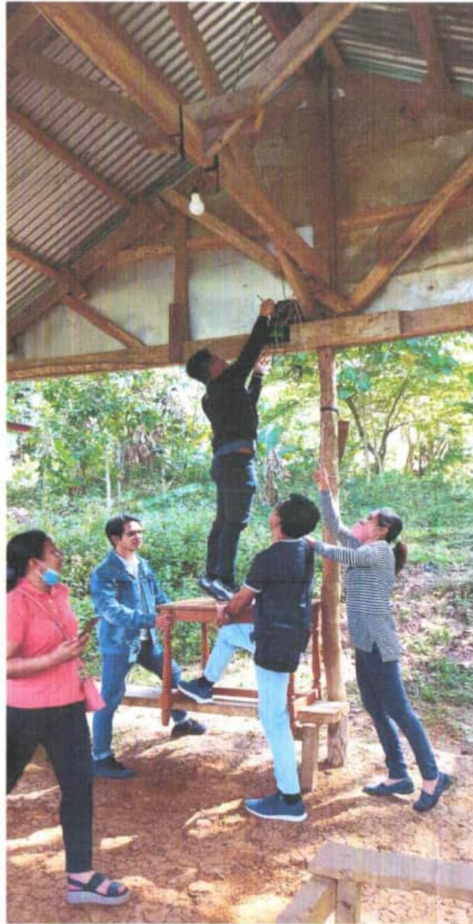
Engr. Harley Tolentino, Faculty extensionist of the EE Department inspects the installed Solar panels.
